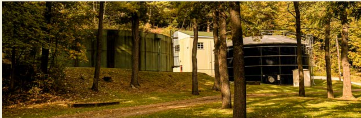
Water Treatment Facility on Dalton Rd
